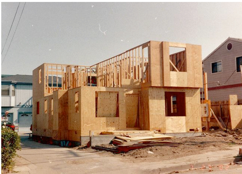
Construction site with Clanco additions, San Bruno, CA
