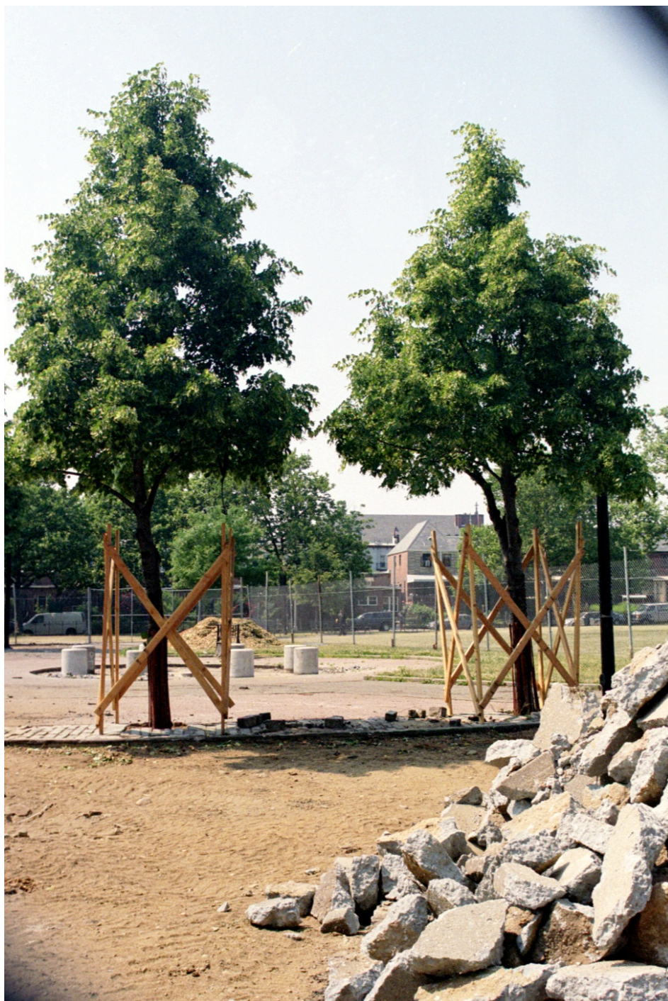
Tree Protectors Installation Brooklyn, NY
